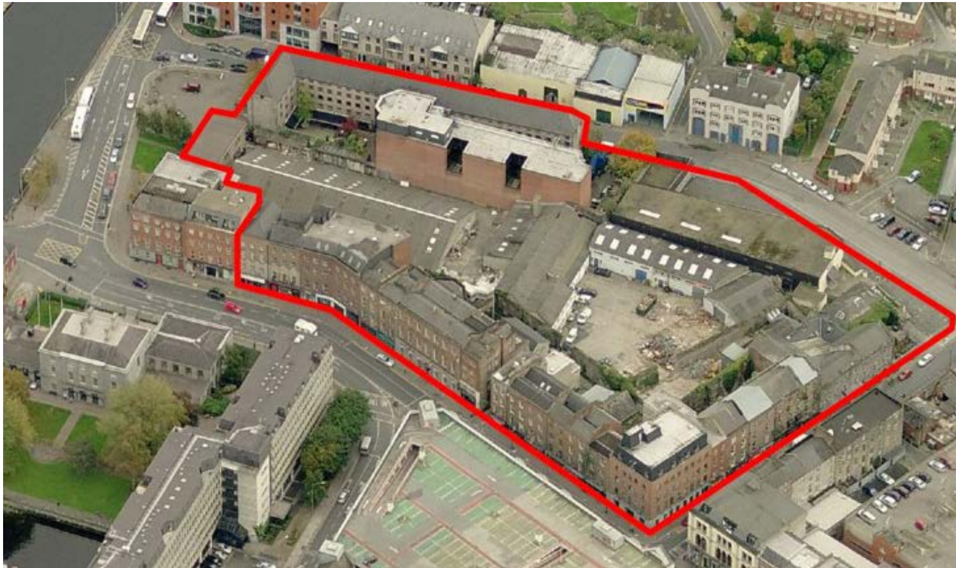
Site Pre-commencement of Works
