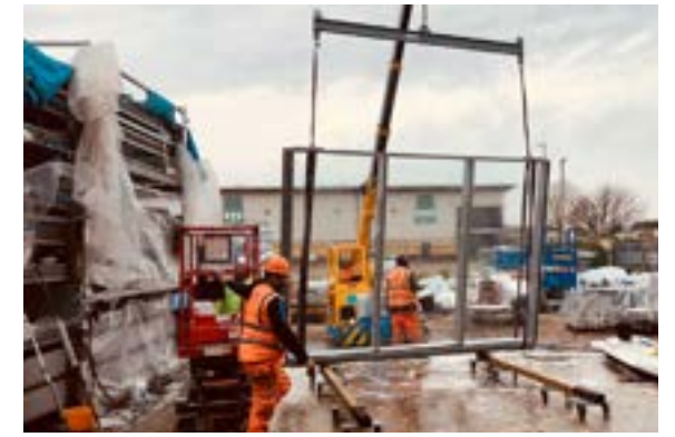
1 Triton Square_ Refurbishment and Reuse of Façade_ ARUP
